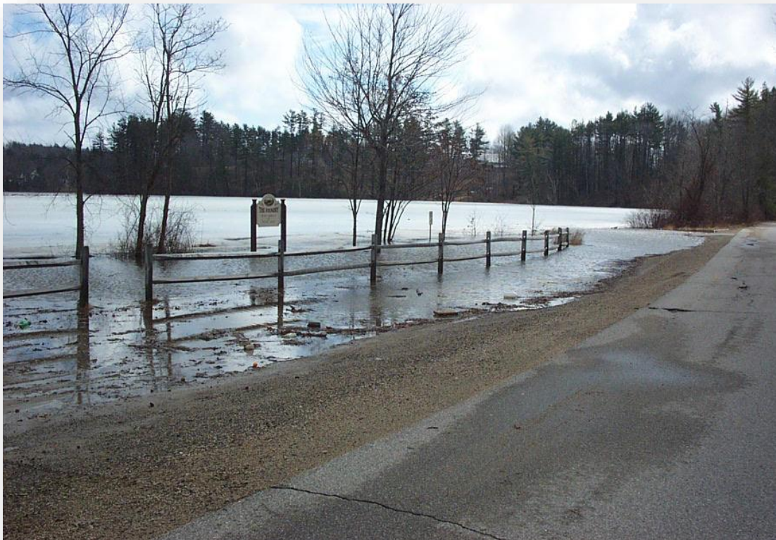
Flooding caused by Hurricane Sandy, 2012 – Rollinsford Police Department
